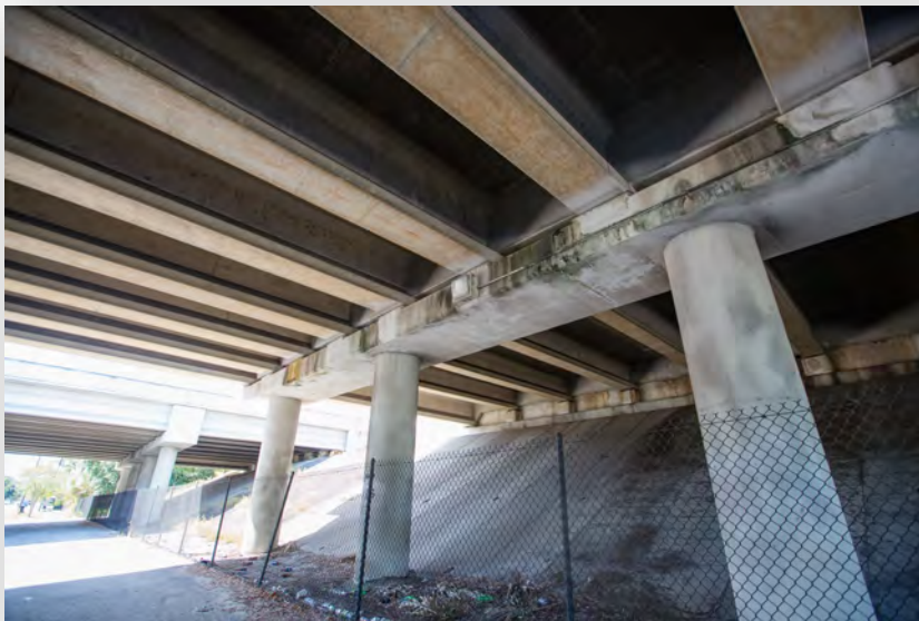
Lighting underneath I-275 overpass
