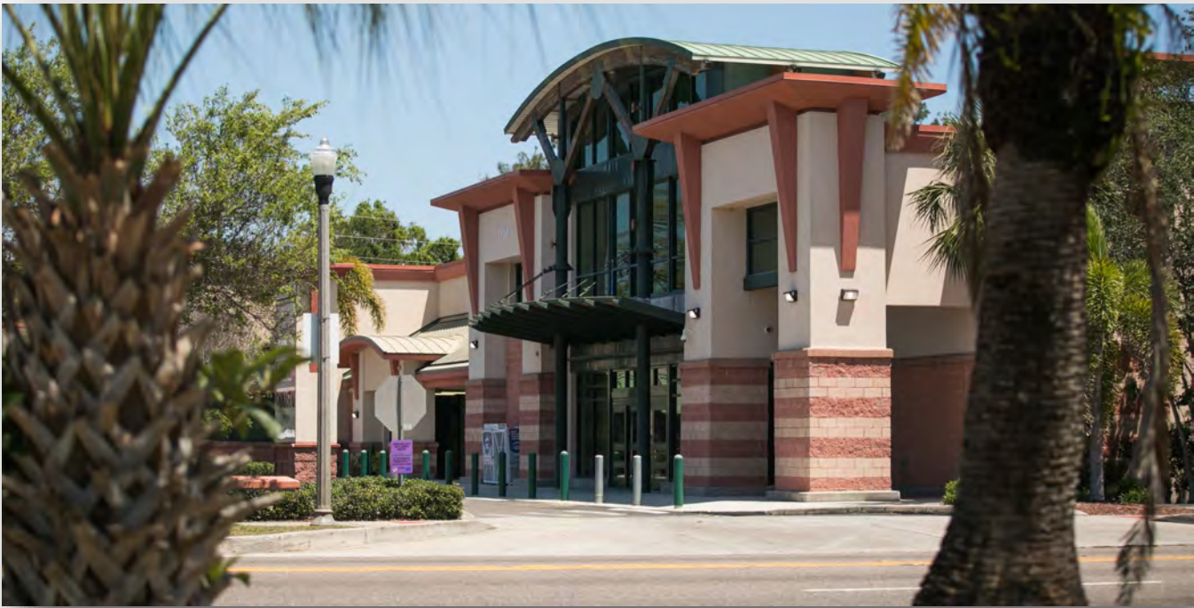
Tangerine Plaza on 18th Avenue South
