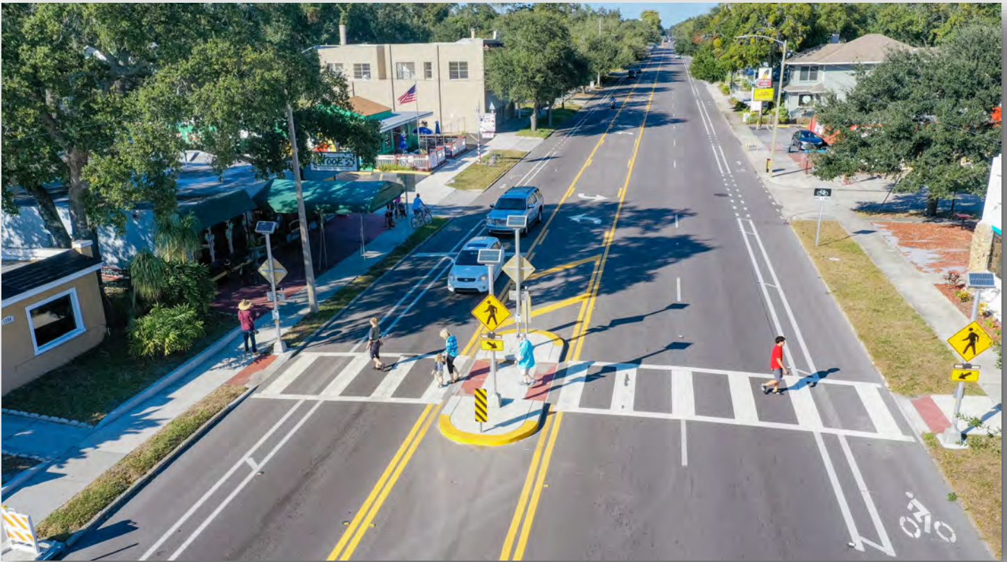
Dr. M.L. King Jr. Street was recently resurfaced with Complete Streets modifications in St. Petersburg
