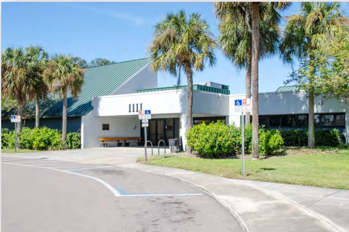
Enoch Davis Center on 18th Avenue South
